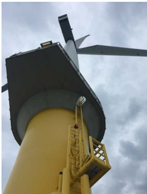
Turbine from waterline.
